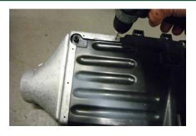
10. Secure in place using pop rivets provided.
