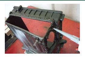
9. Fit aluminium adapter and hold firmly in position. Drill through mounting holes using a 4mm drill.
