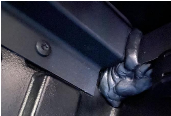
Figure 15 & 16: Window Weld Applied on Inside and Outside of Load Bin at the Front of the Canopy
